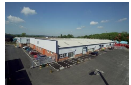
80,000 sq ft refurbished industrial complex in Kent
